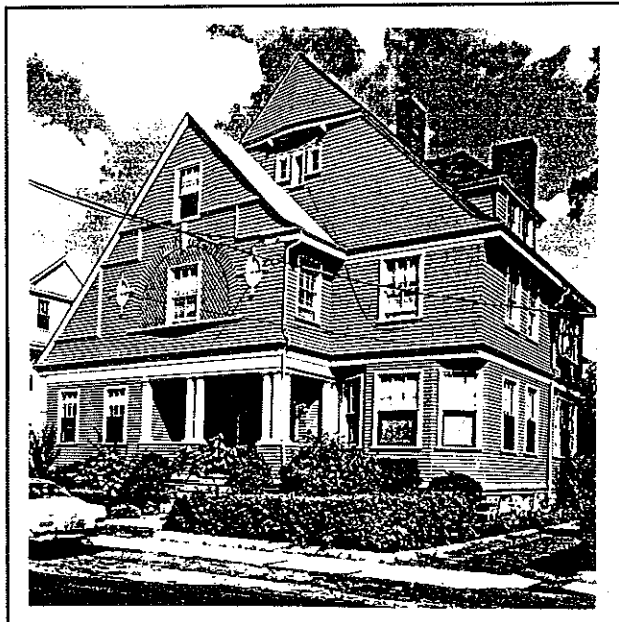
Residence, 5-7 Winter St.
